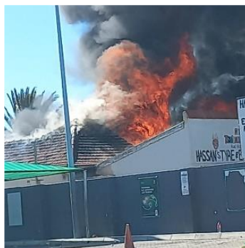
Structural Fire at Hassan's Tyres
