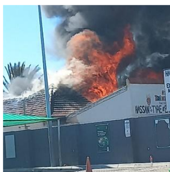
Structural Fire at Hassan's Tyres
