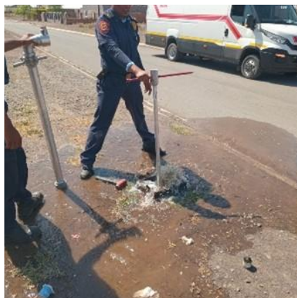
Inspecting fire hydrants in Beaufort West
