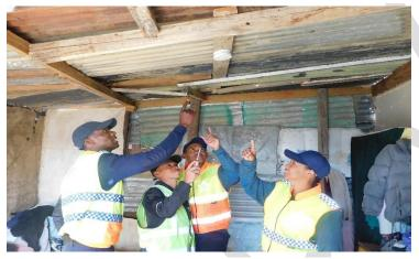
Image 9: Installation of smoke alarms in Laingsburg
