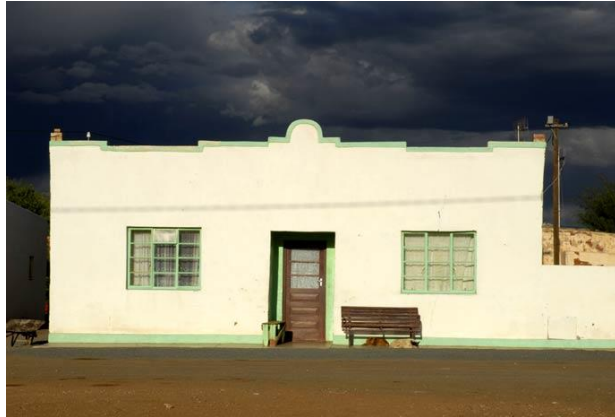
FIGURE 4.11C: TYPICAL KAROO-STYLE ROAD-FRONTING TOWN COTTAGE (source: http://www.findtripinfo.com/south-africa/northern-cape/karoo.html .)
