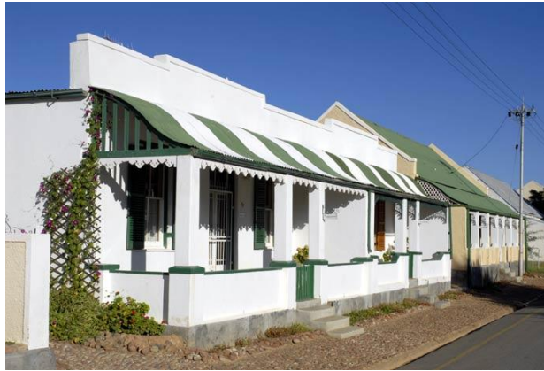
FIGURE 4.11B: ANOTHER TYPICAL KAROO-STYLE ROAD-FRONTING TOWN COTTAGE
